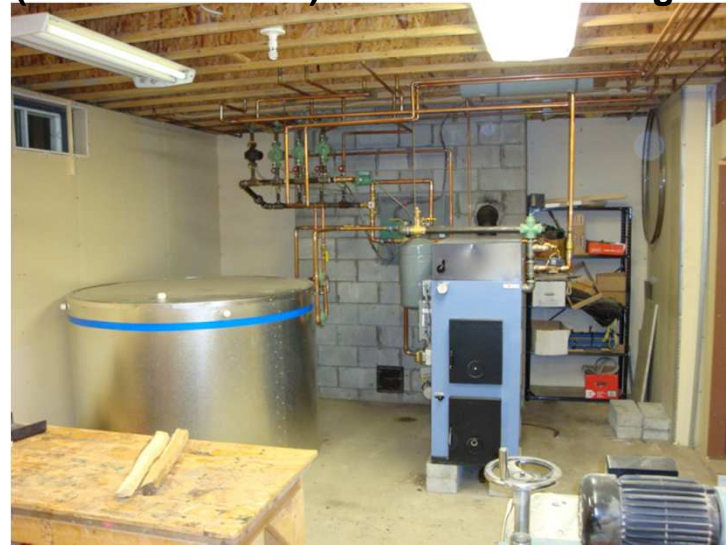
Two-stage, downdraft gasification heater (low-mass boiler) with thermal storage
