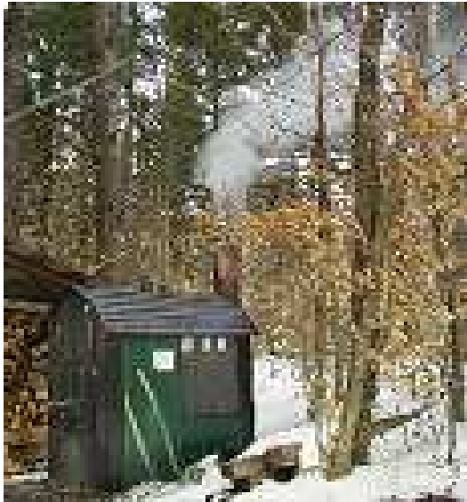
Outdoor Wood Hydronic Heater
