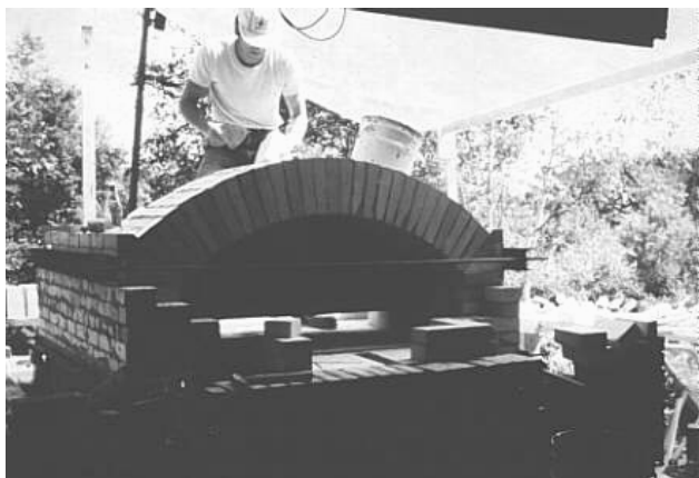
Figure 14 French Commercial Oven. East Wallingford, Vermont, 1984. Firebox is underneath hearth.
