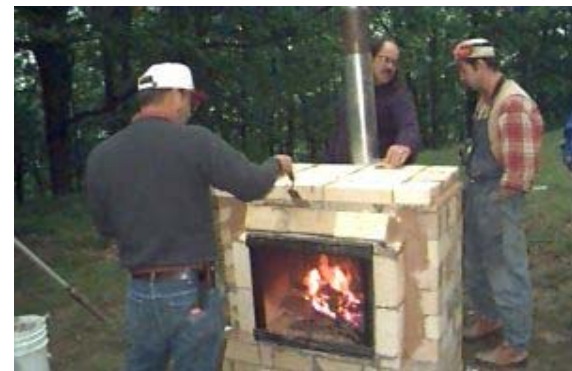
Gary Hart finishes up the burn unit for combustion testing.
