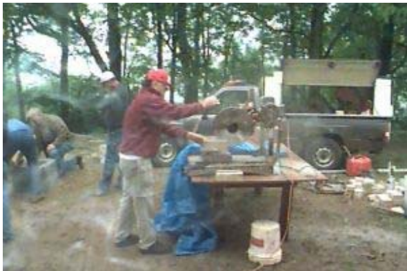
Ben Sotero makes wet dust on the wetsaw
