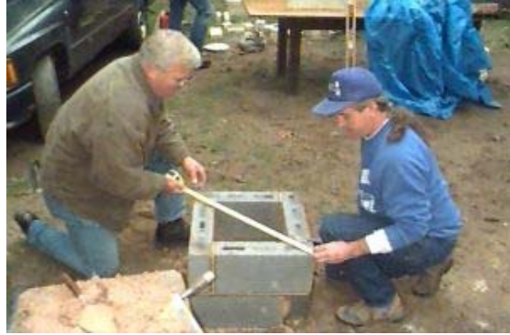
Pat Manley and David Moore square up a base for a certification masonry skills test
