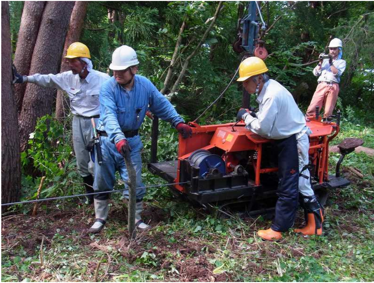
tarring of logging(pulling wire from winch of small tractor).jpg
