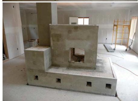
Completed formwork for cast in place concrete bench and capping slabs.
