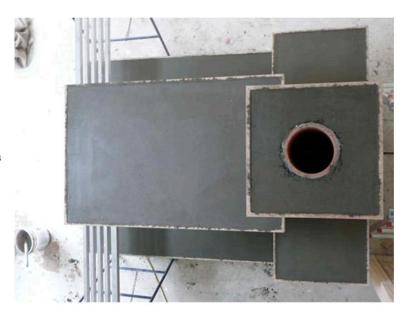
Forms removed showing the freshly cured concrete and the completed rough veneer.
