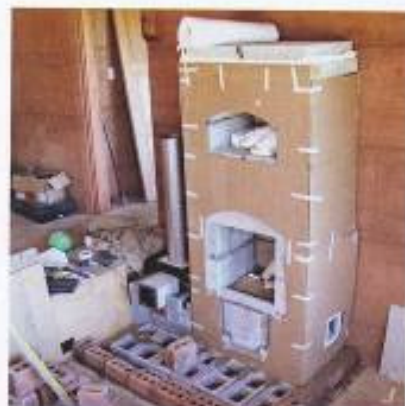
Above: Core completed prior to facing. Left: Facing begun and fire door in place.
