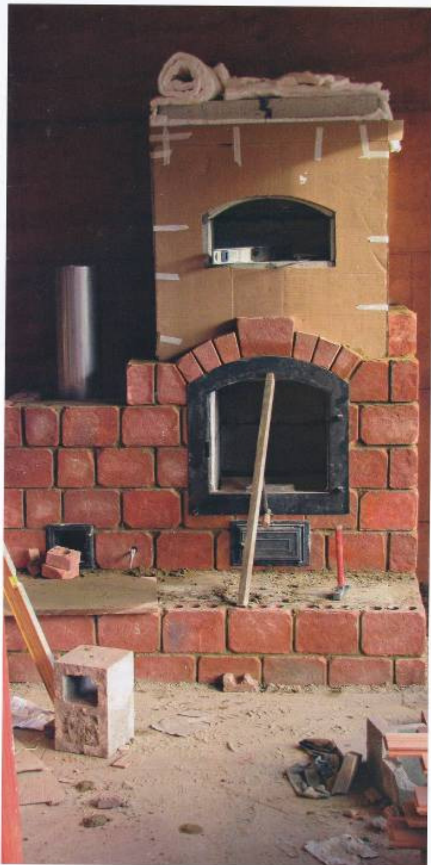
Above: Core completed prior to facing. Left: Facing begun and fire door in place.
